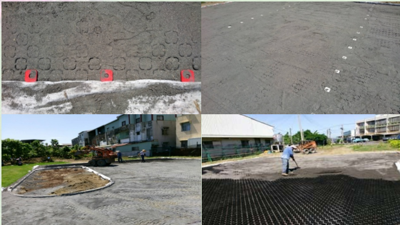
12. Filling the grass grid box with sandy planting medium and labeling.
